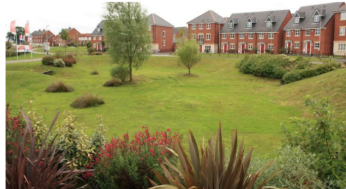
Well landscaped detention basin functional for quantity – Susdrain.
