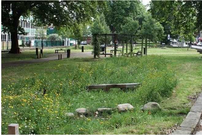
Well landscaped detention basin functional for quantity – Susdrain.
