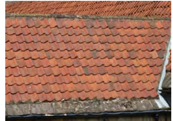
Clay pan tiles and stone slates in a rural context.
